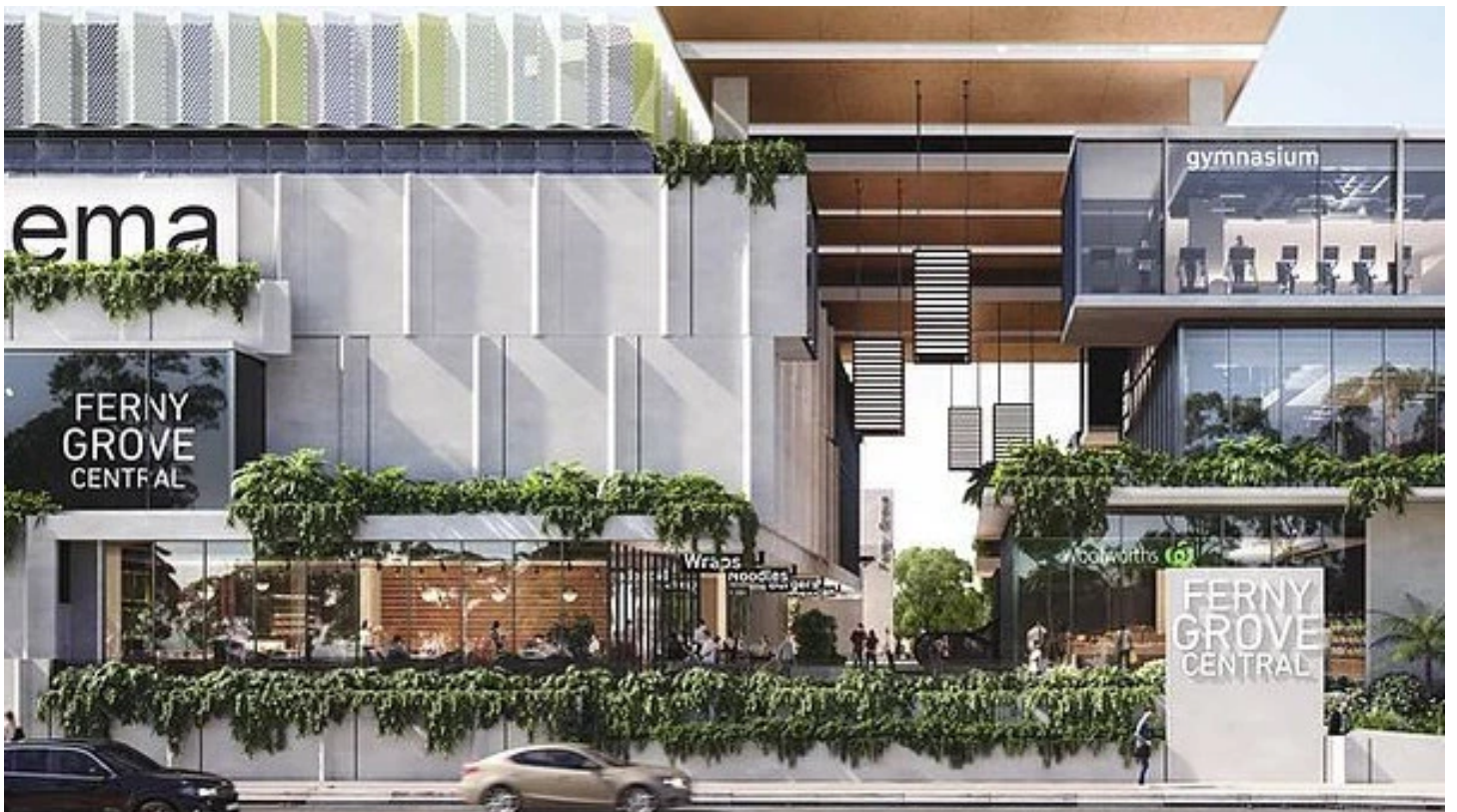
Artists impressions of the $140 million Ferny Grove Central project, construction is now underway. Picture: Supplied.
